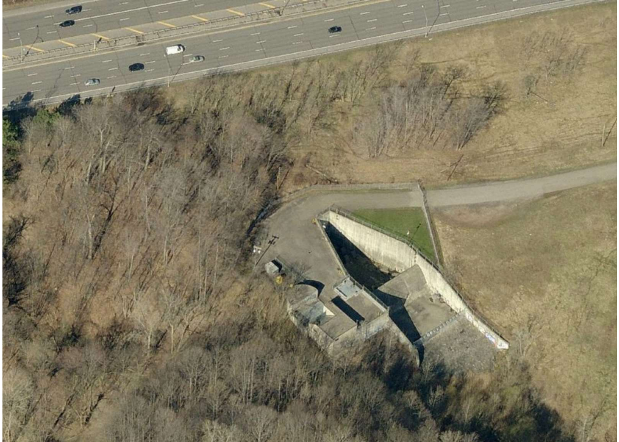
Figure 23: Photo showing the terrain near the Monroe County Pure Waters Culver-Goodman Control Structure. The trail would be between 590 (top) and the Control Structure. Image via rochestersubway.com
