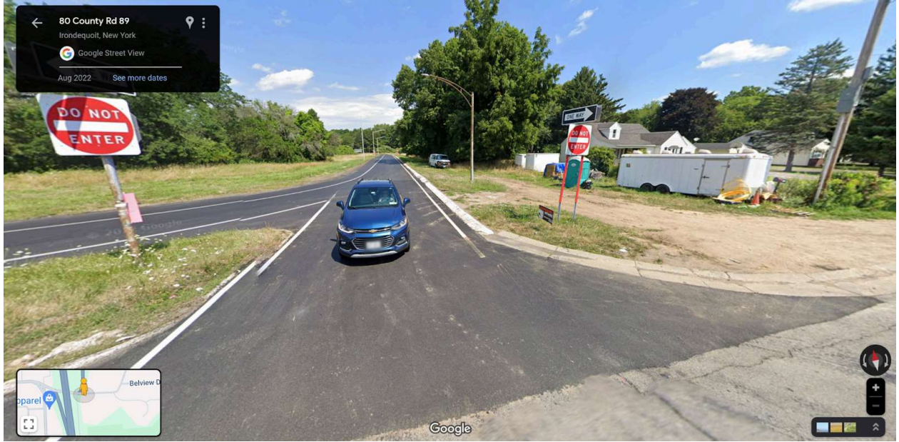
Figure 14: The proposed trail's current southern end at Bay View Road (contiguous with Norton Street). Note the construction equipment and vehicles that are allowed to be stored very close to the off ramp. A trail could easily be built in the space being taken up by that equipment. Image via Google Maps.
